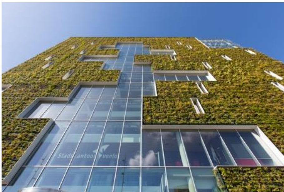
FIGURE 4 NEWLY BUILT CITY HALL VENLO
